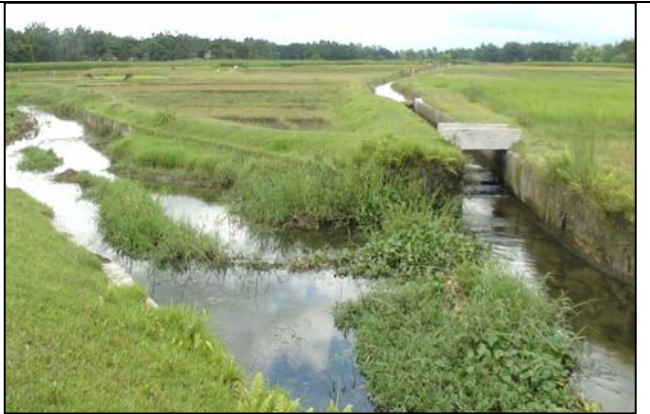
Work done by the irrigation department near the worksite of AAP No. 0704157393/2013-14
